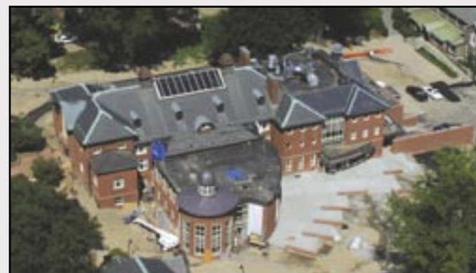
Blanchard Campus Center after remodeling in 2003 (JQS photo)
